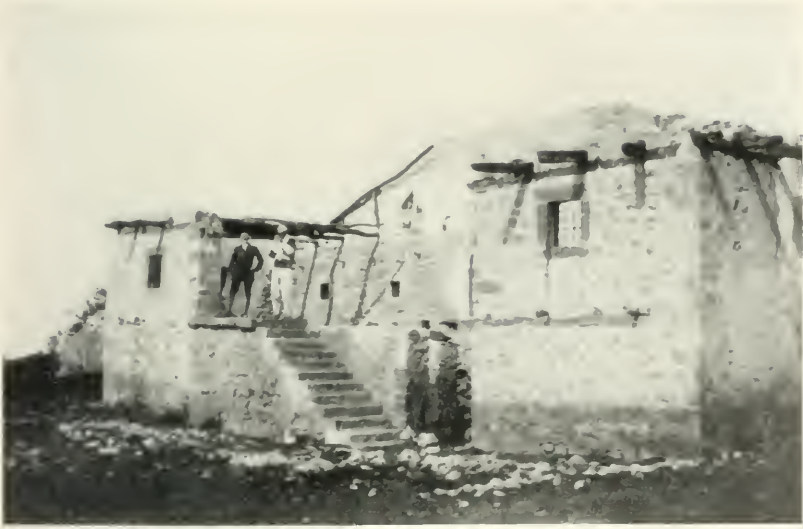
BURNT HOUSE AT GRIZIA.
